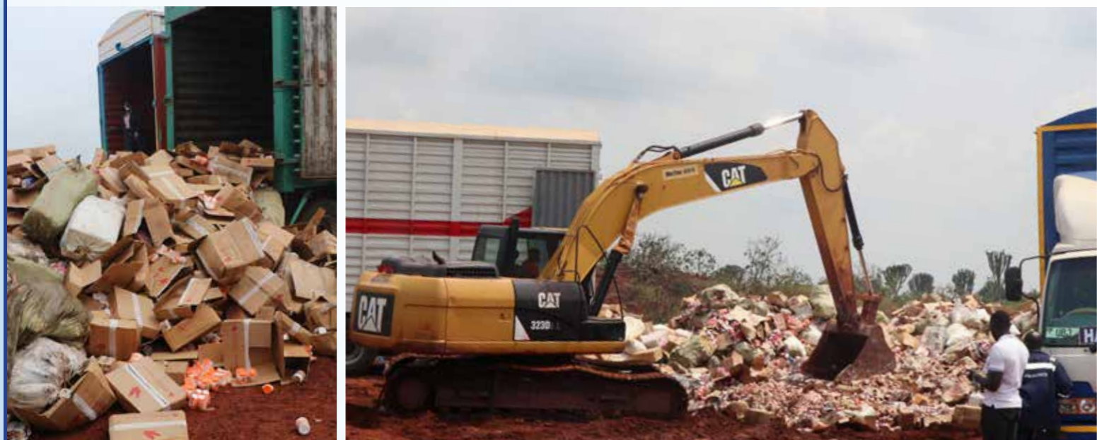
A cross-section of some of the destruction activities in Nakasongola recently.
